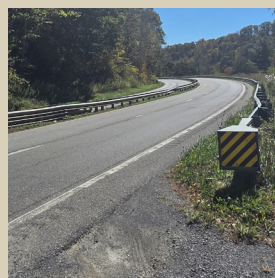
Limited Sight Distance
