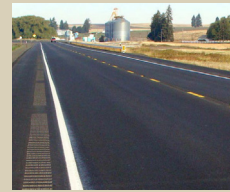
Centerline and Edgeline Rumble Strips ($)
