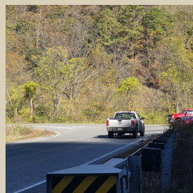
Limited Sight Distance
