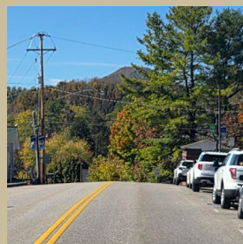
Limited Sight Distance
