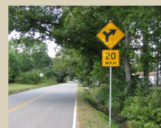
Curve Warning Signs with Advisory Speeds ($)
