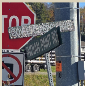
Lack of Needed or Compliant Signs
