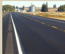
Centerline and Edgelines Rumble Strips ($)
