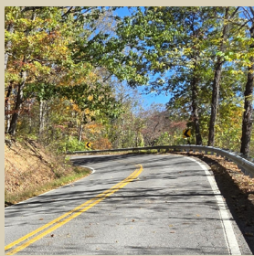
Limited Sight Distance
