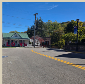
Limited Sight Distance
