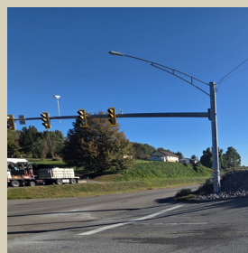
Limited Sight Distance
